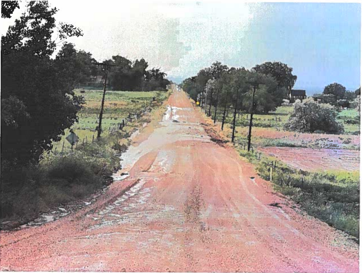
49 th Street West of PUD Entrance
